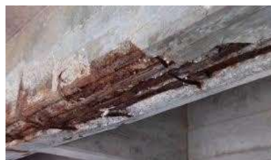
Fig.22 effect of corrosion in reinforcement
